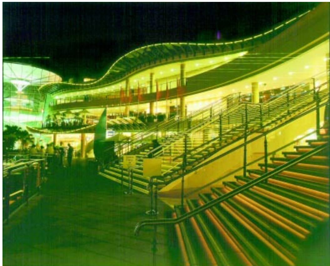
Fibre optic awning rods
